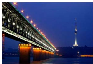
Yangtze River Bridge
